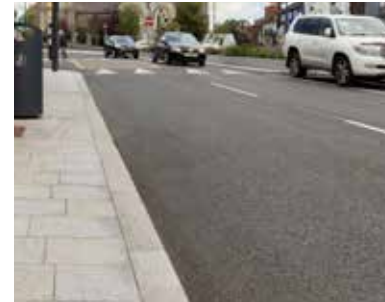
Asphalt Surfacing / Granite Kerbs
